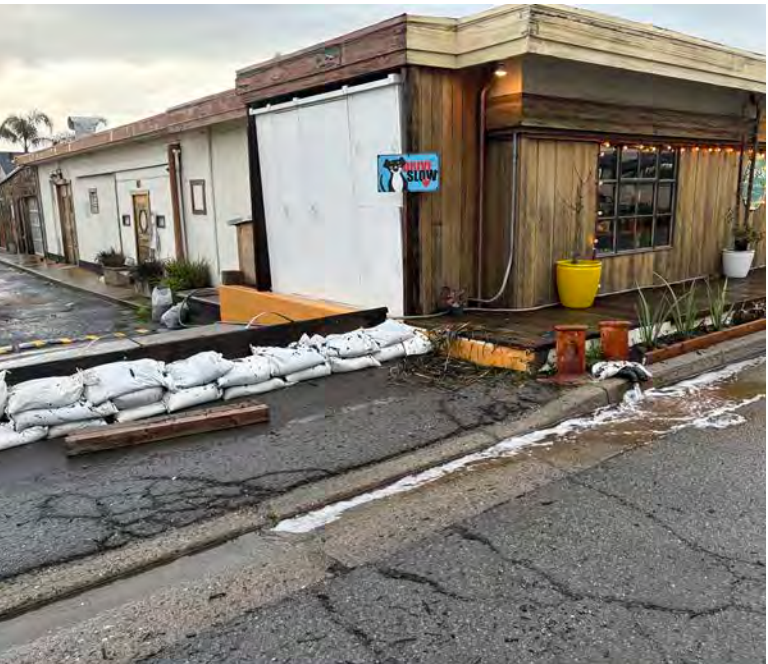
Sand bag protection on Gate 5 Road
