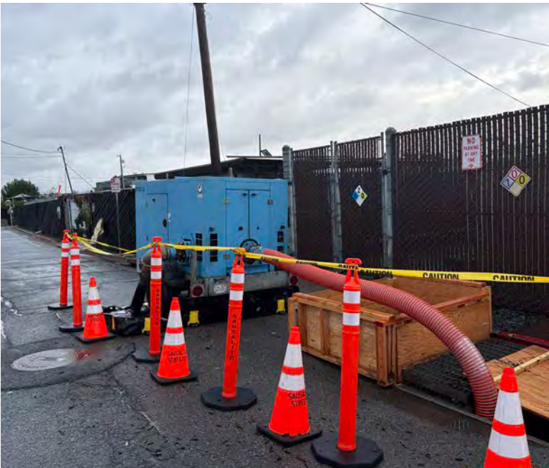
City's temporary pump installation on Gate 5 Road
