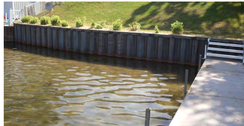
Seawall made with vinyl or concrete
